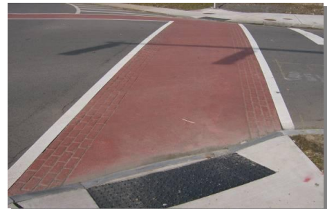
Example of a colored and textured crosswalk
