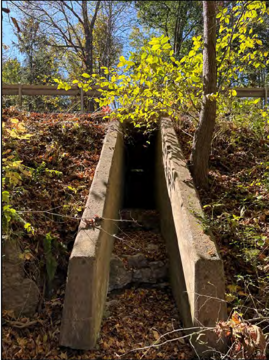
Photo 23. Culvert with extended wingwalls passing under Taughannock Blvd
