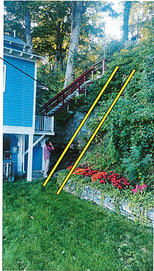
VIEW OF APPROXIMATE TRAM TRACK LOCATION
