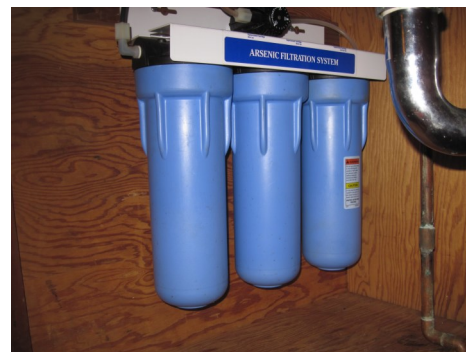
Figure 4.—Photographs of a ferric adsorption point-of-use filtration system installed beneath a kitchen sink.
