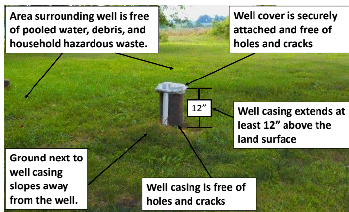
Figure 1: Photo of a properly constructed well.
